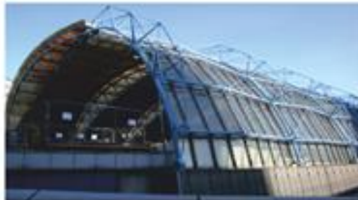
WATERLOO INTERNATIONAL TERMINAL
