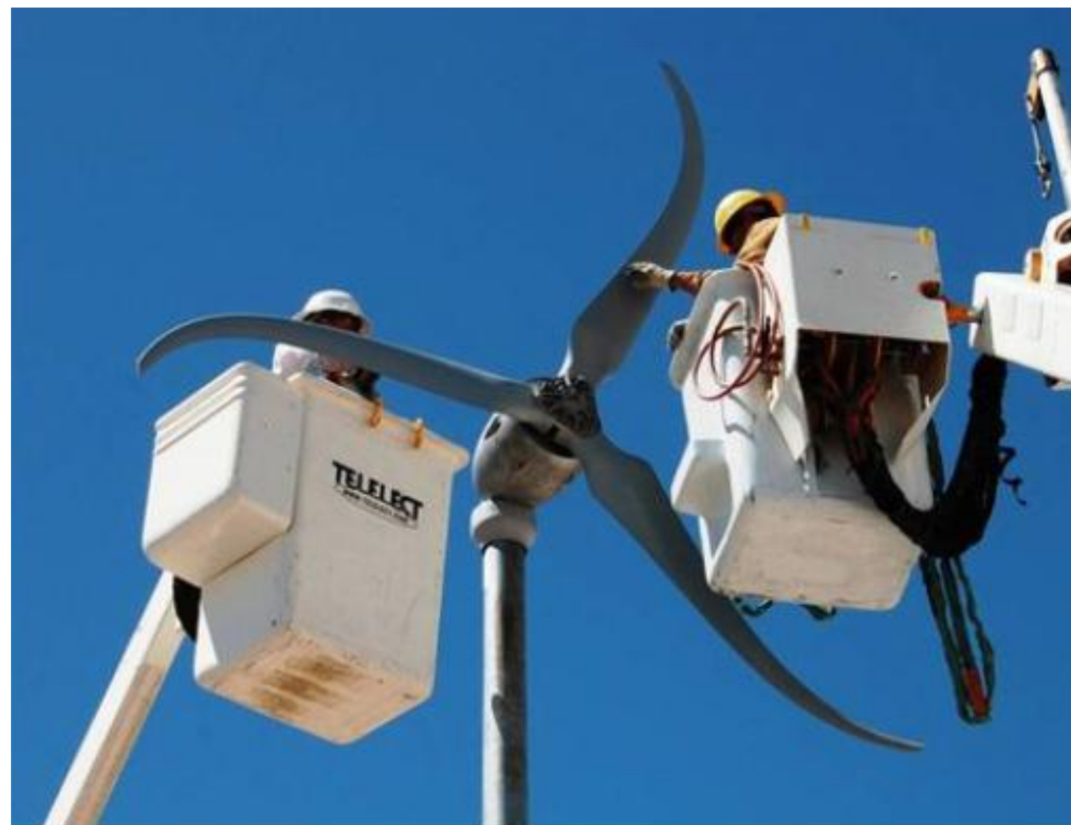
Photo from Chris Brooks, NREL 16743
