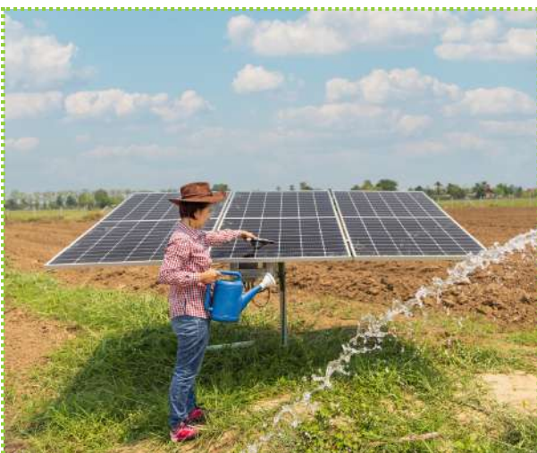
solar panel system
